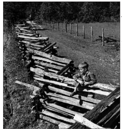
An American invention, the worm (or zigzag) fence was easy to build because it required no posts: St. Augustine County, Texas, 1939.
